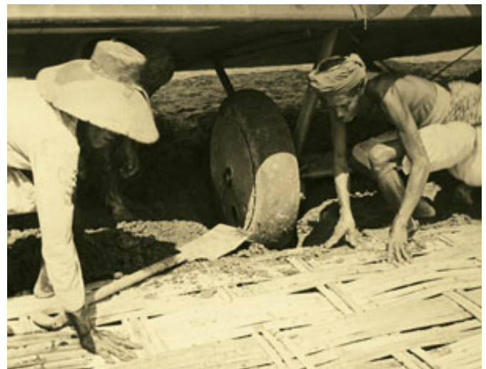
A makeshift runway made of bamboo mats enabled the Vimy to take off from Surabaya, Java. Courtesy of National Geographic Society
